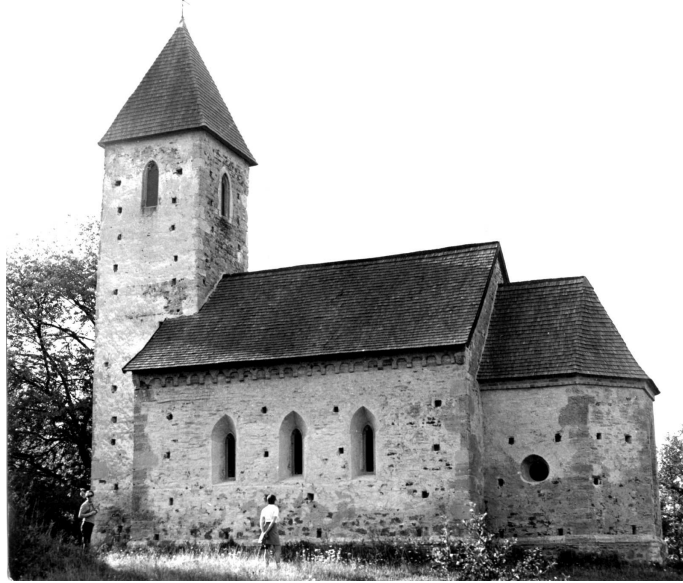
Figure 1: Southern view of the church.
